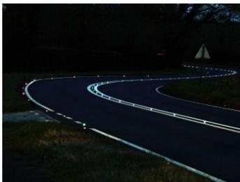
The SolarLite solar-powered road stud, made in Bicester, Oxfordshire, is now in use in 120 UK locations and 20 countries overseas. The product has built-in light emitting diodes which can give drivers up to 900 metres of visibility after dark, ten times more than a conventional 'catseye' containing a simple reflector.
